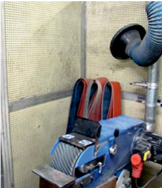
Figure 13 Movable acoustic screen in a foundry
